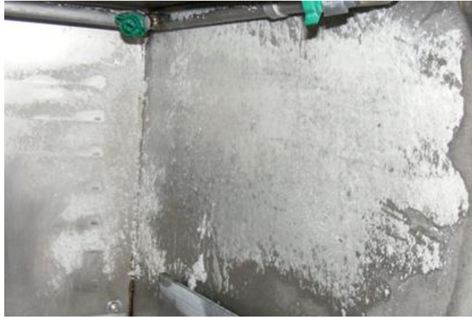
Prior to installation
