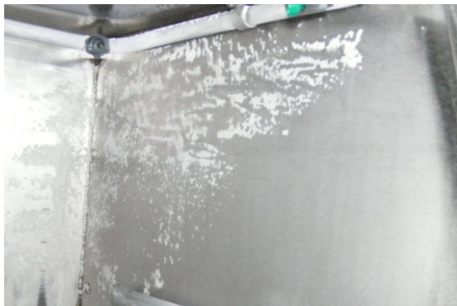
6 months after installation
