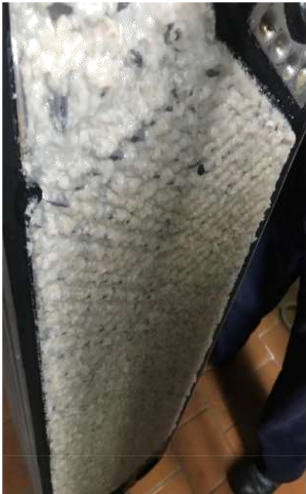
2018.06.05 Before installation of Hydroflow device
