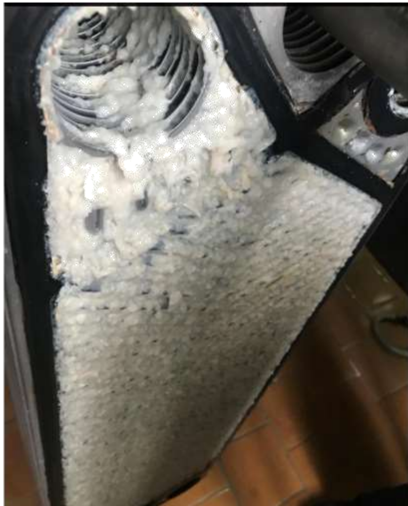
2018.06.05 Before installation of Hydroflow device
