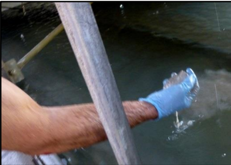
Scale which was removed is settling in the sump as fine silt
